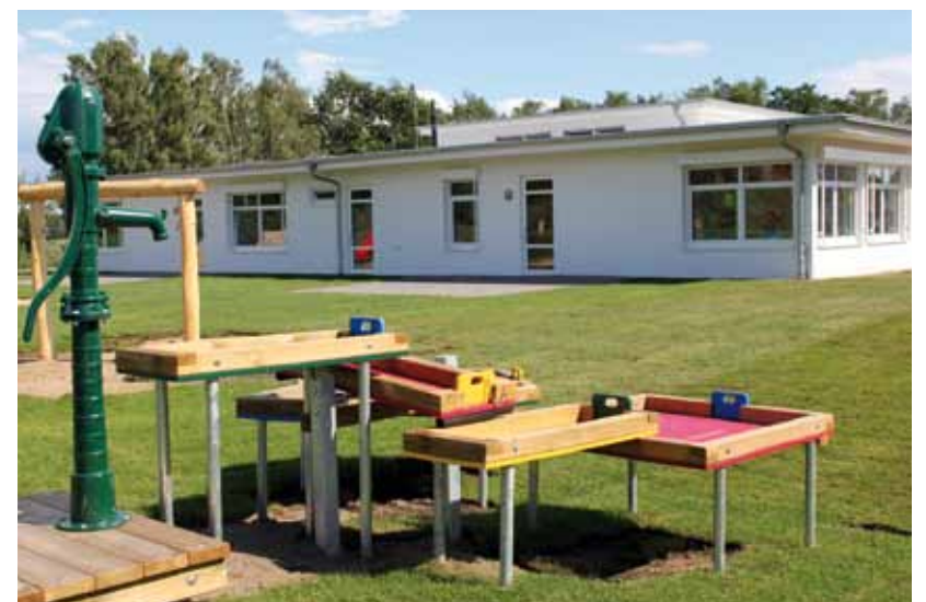
day-care centre Robin HuD
